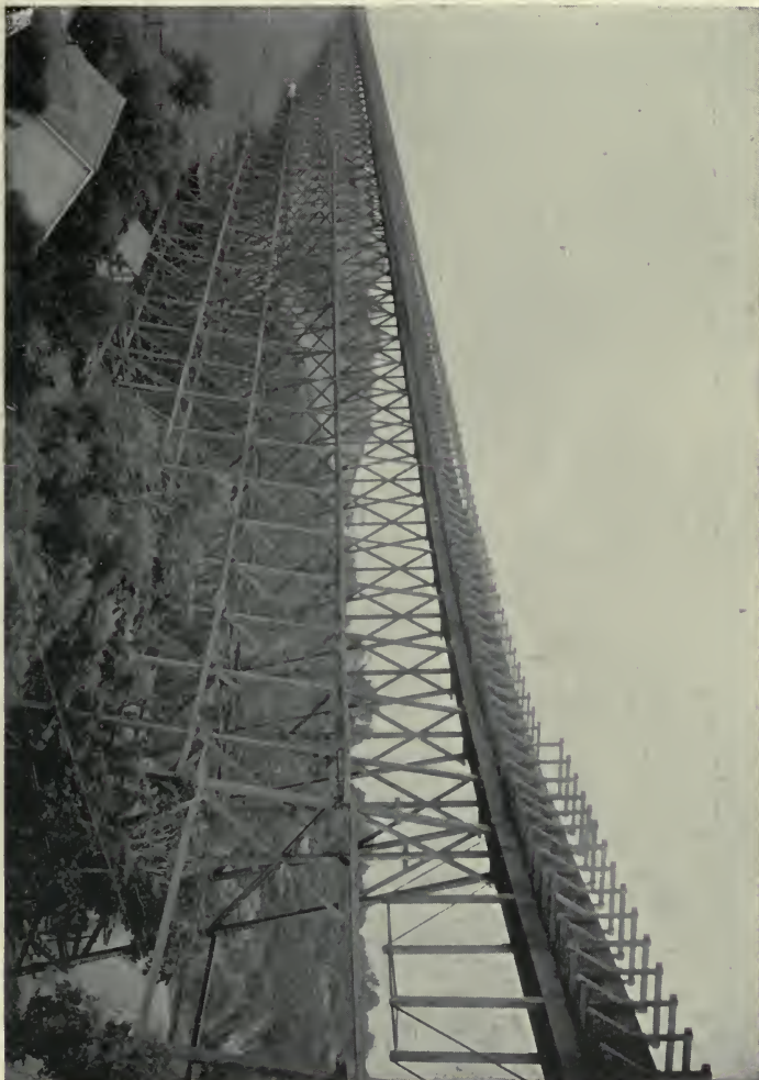
IRRIGATION IN SAN JOAQUIN COUNTY A Flume 95 feet high and 2,700 feet long
