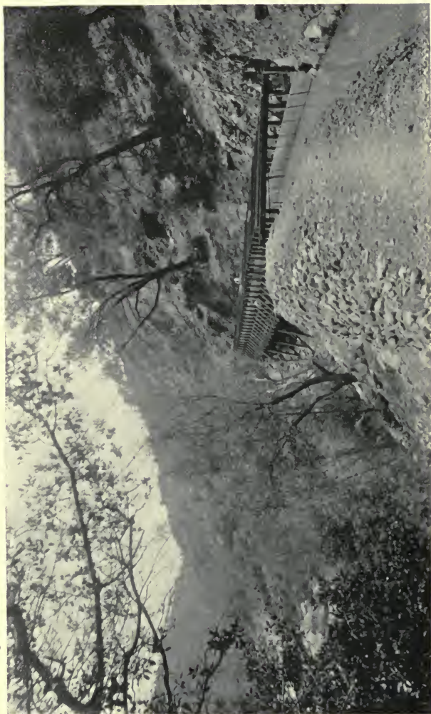
IN THE MOUNTAINS OF SAN JOAQUIN COUNTY Bringing Water to the Plains in a flume ten feet wide and seven feet deep
