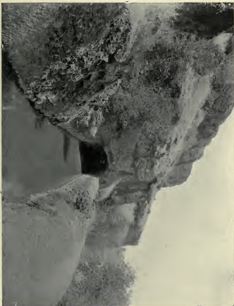
IN THE CAÑON OF THE STANISLAUS RIVER A Tunnel 1037 Feet Long Through Solid Rock, Carrying Water for Irrigation
